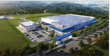
Completed and launched operations at the new Cheongju Power Distribution Campus
